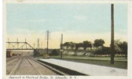
Approach to Overland Bridge, St. Johnsville, N. Y.
