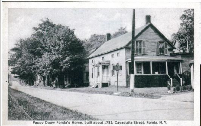
Pappy Douw Fonda's Home, built about 1781, Cayadutta Street, Fonda, N. Y.
